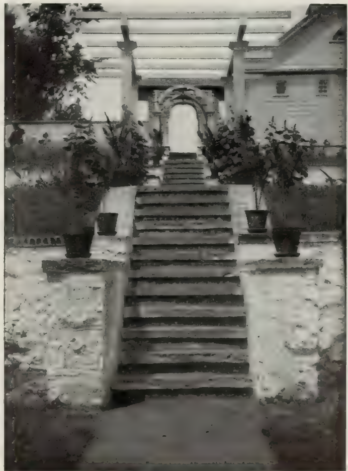
TERRACED STEPS IN GARDEN OF THE HOUSE FOR FRANK SQUIER, ESQ. GREENWICH, CONN.
